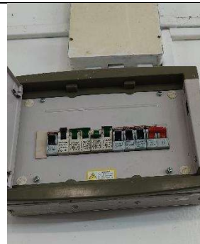
Photo: IQAC DB (Admin Bldg. GF)
